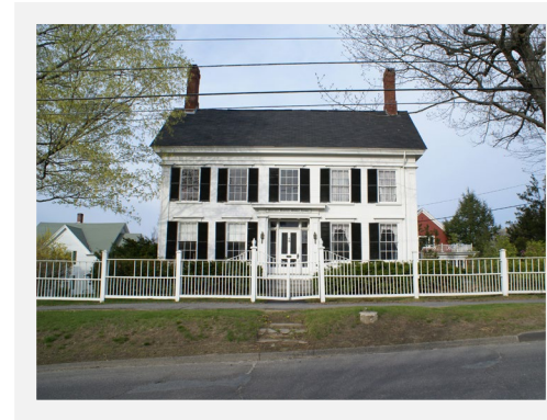
Harriet Beecher Stowe House
