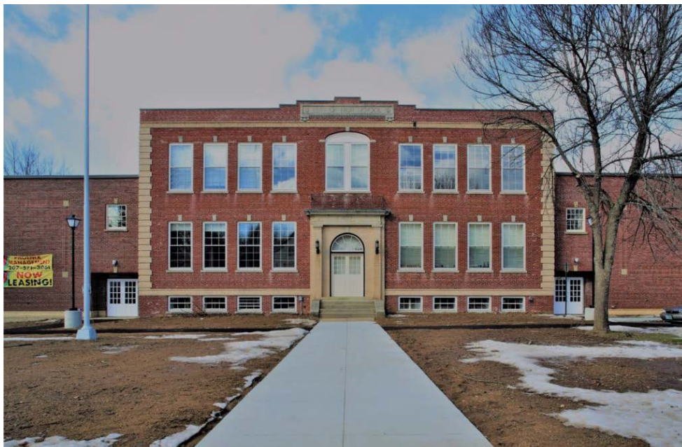
Sullivan School Apartments, Berwick
