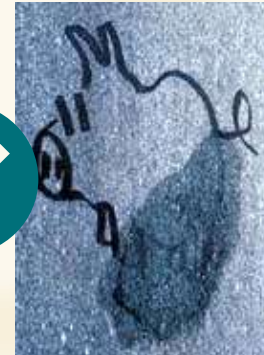
Graffiti removed from historic building with poultice
