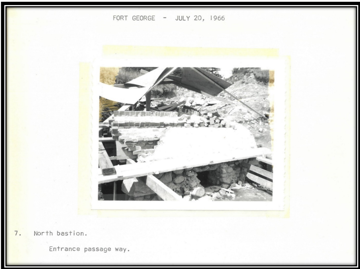
Figure 4-14. Photograph of the 1966 State of Maine Park Commission-funded restoration of the stone and brickwork of Fort George, in the north (northeast) bastion of the fort (Files of the Maine Bureau of Parks and Lands).
